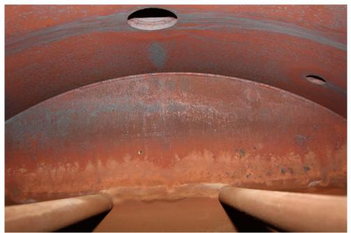
Fig 2. Boiler waterside looking towards the front tubeplate.
